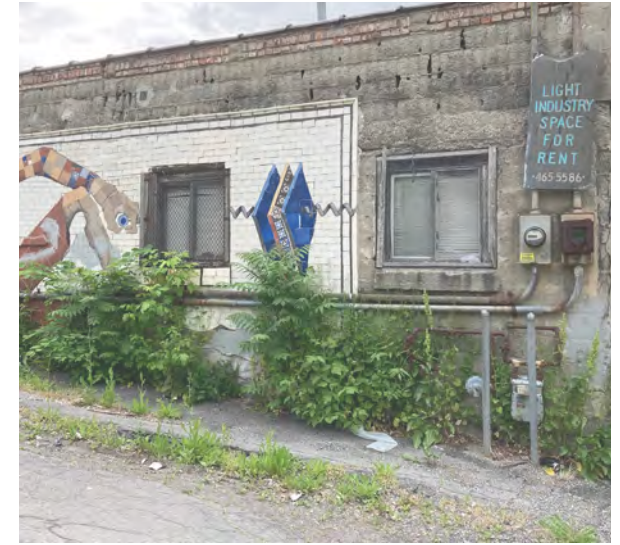
former Tile Factory existing conditions
