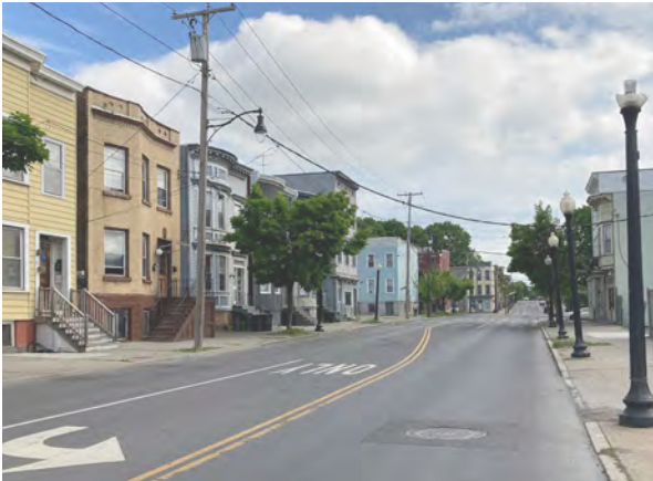
existing conditions: Henry Johnson Boulevard
